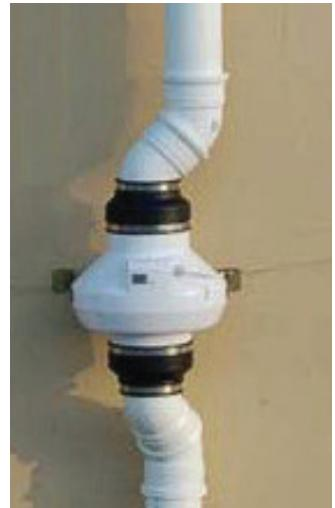
Airflow under suspended floors also can be increased by installing vents. This method has been proven effective on radon levels of up to 700 Bq m<sup>3</sup> in some cases and can be improved by adding fans to create greater movement of air.
