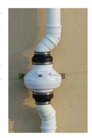
Sump fans can be installed externally or internally.
